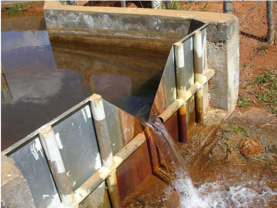
Figure 6.4 Spillway of a small dam in the Buriti Vermelho catchment
